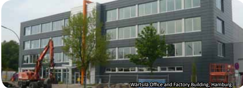
Wärtsilä Office and Factory Building, Hamburg
